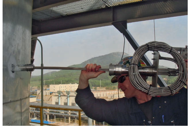
WIKA/Gayesco service team employee installing a Radial Tap™
